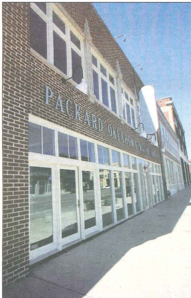
The building is the new home of Accel Financial Staffing.
